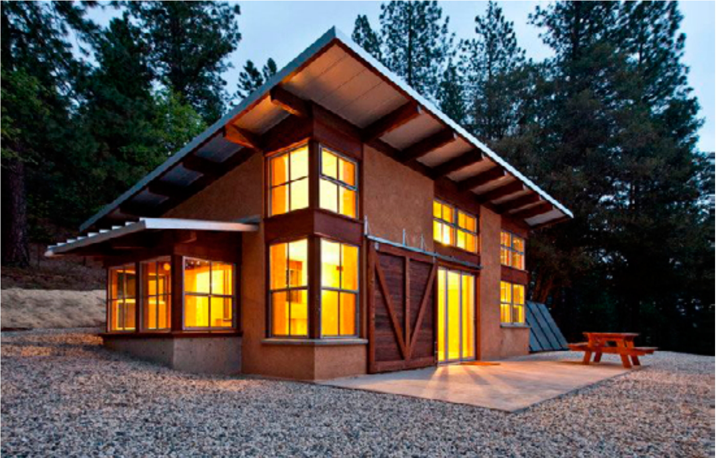
Designed for California's wildfire country, this 872-sq.-ft. cabin is a hybrid straw-bale home. That means that while some of the walls are conventionally built with dimensional lumber and the roof is made of SIPS, the rest is built with straw-bale construction techniques.
