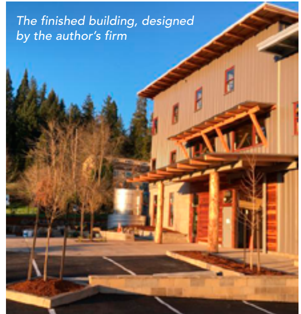
Insulating a stick-framed, mixed-use building with straw bales
