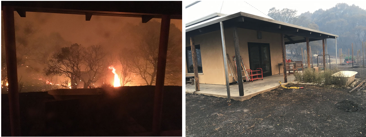
fig. 5. Redwood columns salvaged from a prior fire frame the conflagration; charred but did not ignite.
