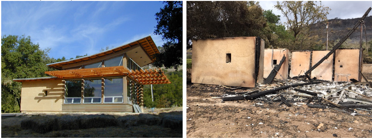
fig. 6. Napa Studio burned in the Atlas Fire; strawbale walls burned after the roof above was breached.
