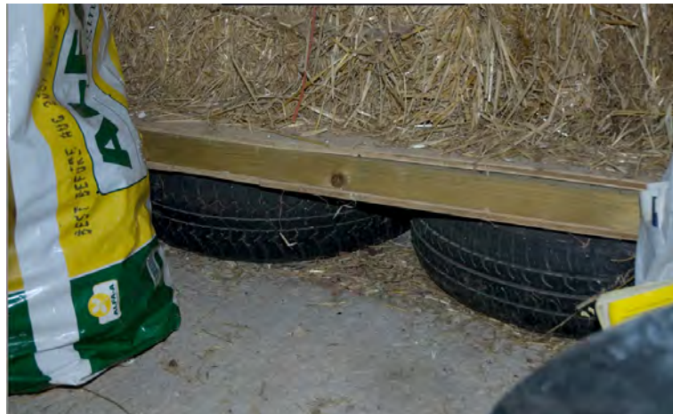
Fig.A4 Straw supported on tyre wall.
