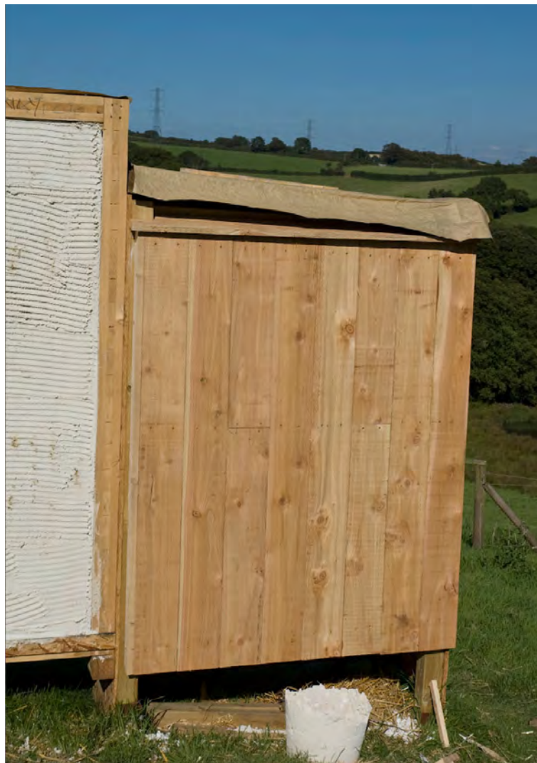
Fig.91 Panel at Liskeard with timber cladding
