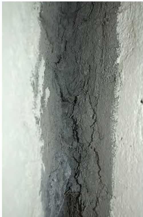
Fig.A28 Meeting of two walls at Footprint Visitor Centre
