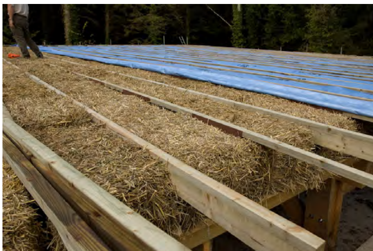
Fig.A18 Straw bales used in roof of sawmill
