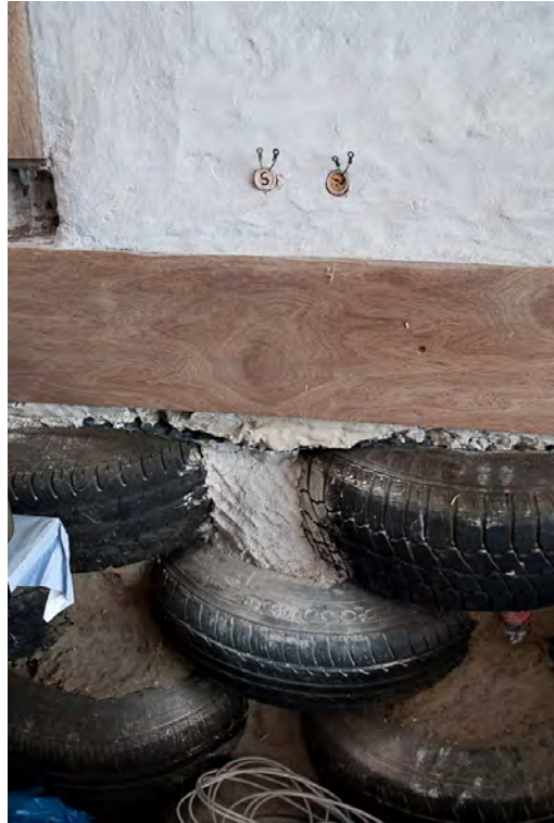
Fig.A31 Rammed earth tyres used as retaining wall
