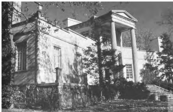
Fig.9 The Burritt Mansion. The first two storey framed straw bale house (1936) From Steen et al. (1994).
