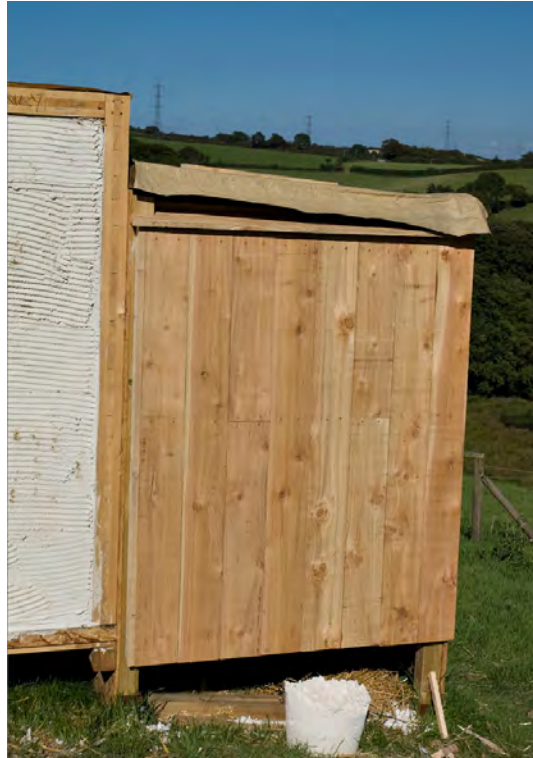
Fig.A14 Timber cladding on panel
