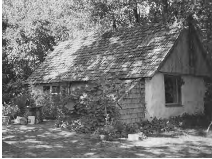
Fig.10 The Hay House, built in 1974. From Lacinski and Bergeron (2000).
