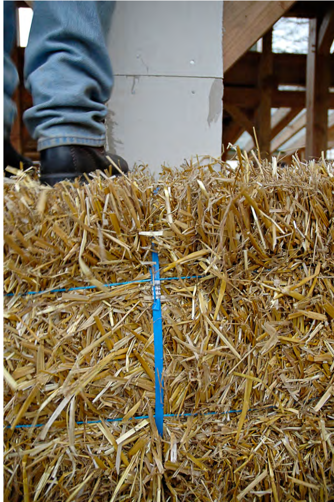
Fig.66 Bale laid on edge, held against post with polypropylene strapping.
