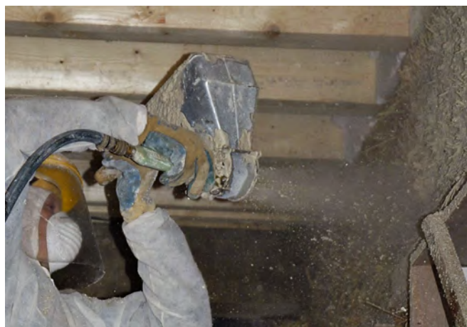
Fig.65 Using a compressed air render gun to apply the lime render
