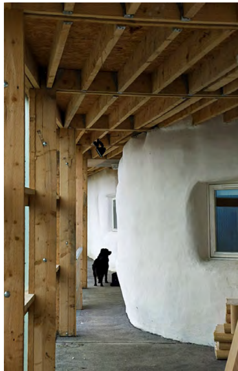
Fig.A16 Straw bale wall of Hedgerow House
