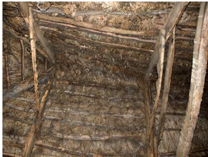
Fig.4 Five hundred year old smoke blacked thatch at Uppacott
