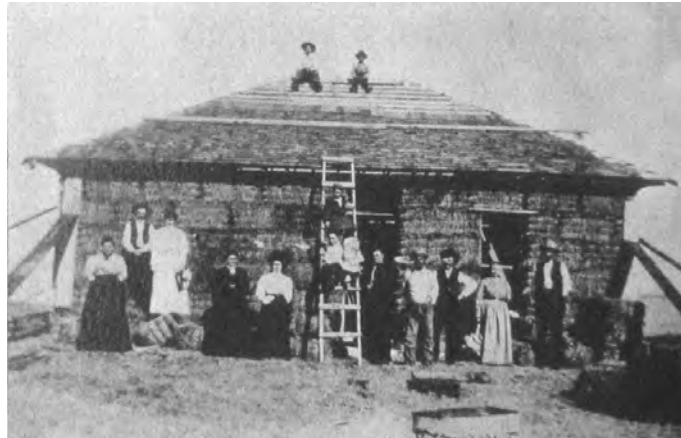
Fig.7 Contemporary photograph of the Simonton House, Purdum, Nebraska during construction in 1908. From Lacinski and Bergeron(2000).
