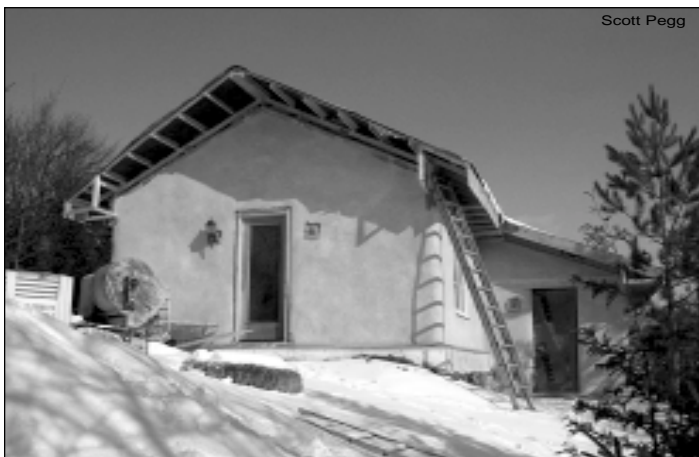
Scott Pegg's building is the first code-approved, loadbearing structure to use earthen plasters in "strictly-by-the-book" Ontario.
