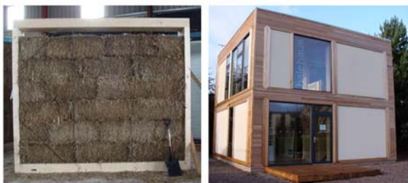
Figure 4 ModCell panel under construction in a 'flying factory' (left) and the completed prototype house at the University of Bath campus (right).
