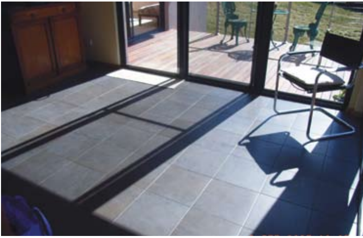
Fig. 1 Concrete floor and dark tiles serves as thermal mass in this house
