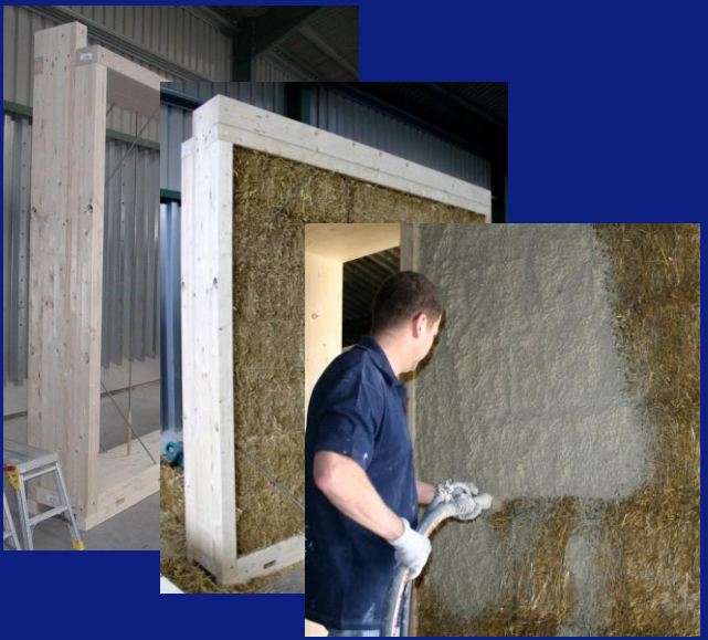
ModCell panel construction
