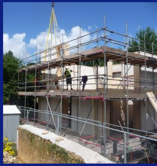
Construction of BaleHaus at Bath
