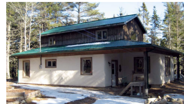
Lime plaster final coat (215)
