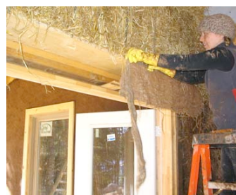
Covering wood with burlap
