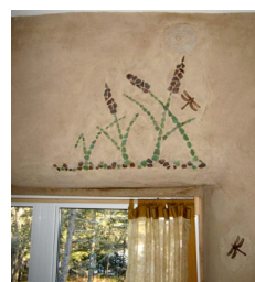
Repaired plaster with inlay art (215)
