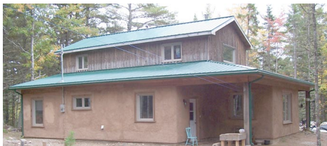
Earth plaster ground floor, board and baton second floor.
