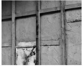
Fig 7. Battens fixed to the horizontal 'ladder' and single coat of lime render applied.
