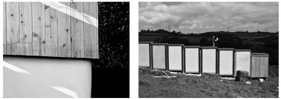
Fig 1(Right). External wall of Totnes house showing use of a vented timber rainscreen and plain render on the same elevation Fig 2(Left). Straw bale panels protected with different renders including, on far right, panel finished with timber rainscreen
