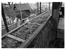
Fig 6.'Ladder' made from 38x38mm batten, laid on the second course of bales, provides a valuable fixing point both on the inside and outside of the finished wall.
